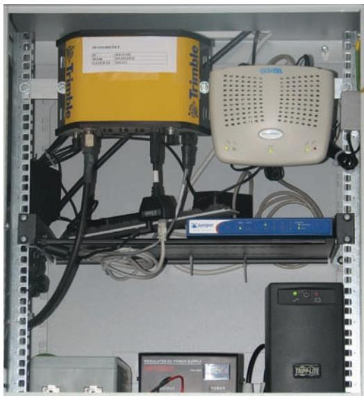
Picture 3: Cabinet with the GPS receiver
